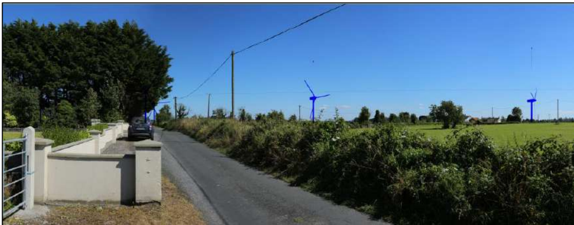
Plate 13-14 Photowire image PW-F from the west at 1km showing partial visual screening and comparatively more modest perceived scale of visible proposed turbines than what is shown in VP14
